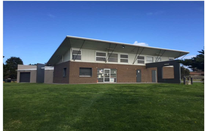
Figure 1: Lawson Poole Reserve Pavilion – pre-redevelopment
