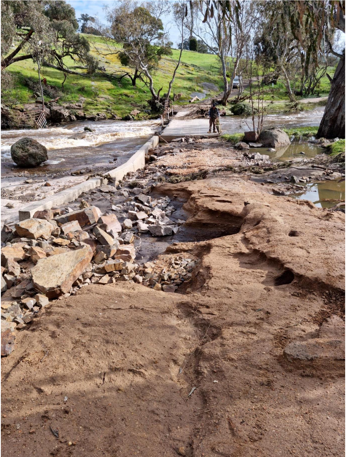
Flood Damage at Hughes Creek Bridge, Ponkeen Creek Road, Tarcombe
