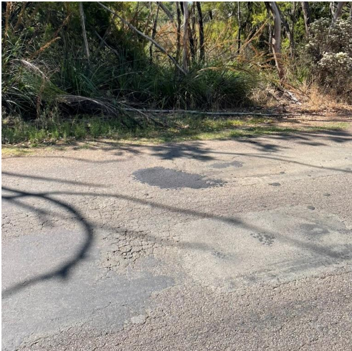
Figure 1 – Underground aquifer as evidenced by repeated potholing and lush vegetation (Boundary Hill Road, Boho South)
