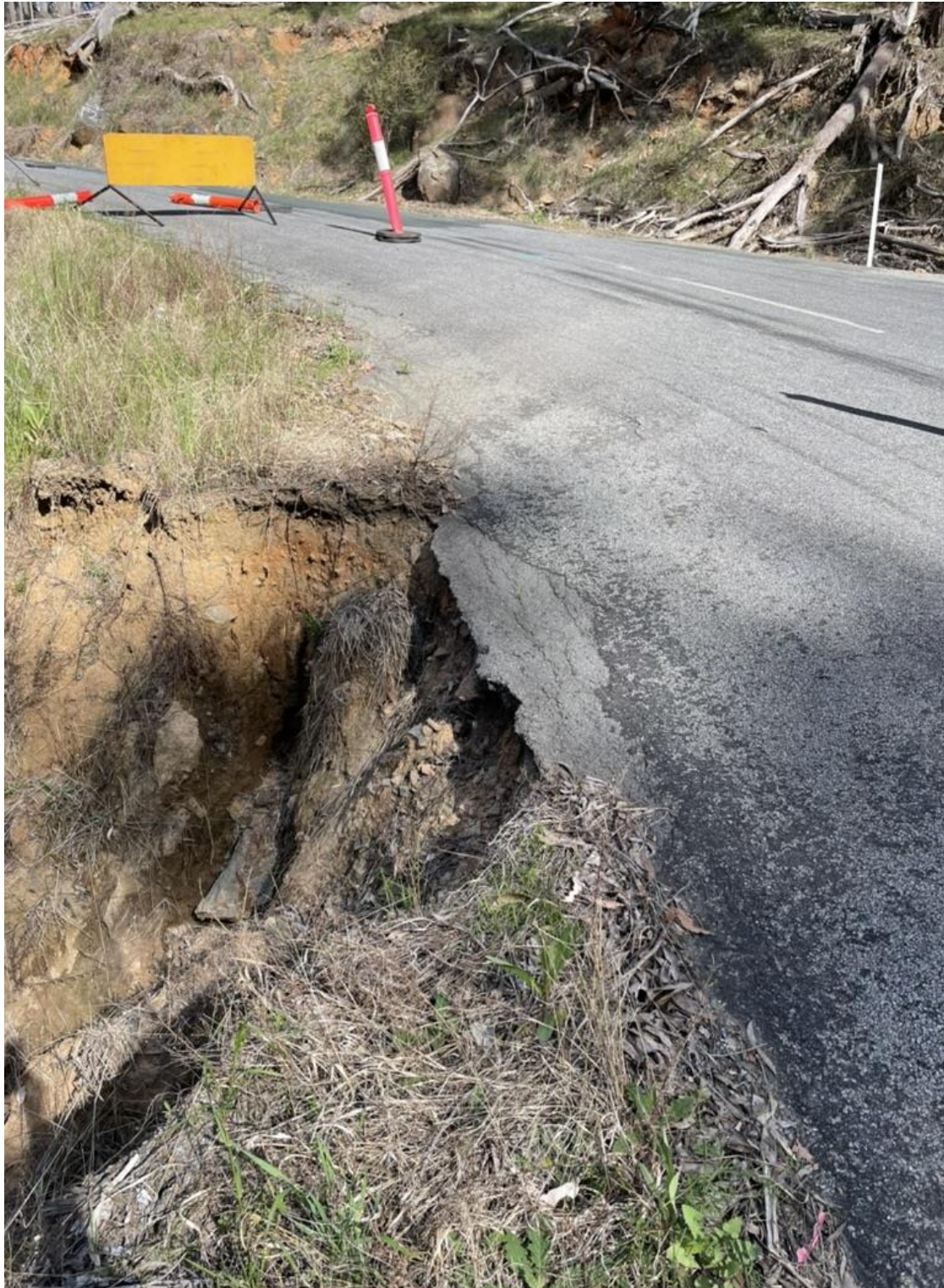
Figure G(i) – Erosion damage due to water sheeting from steep gradient at Harrys Creek Road
