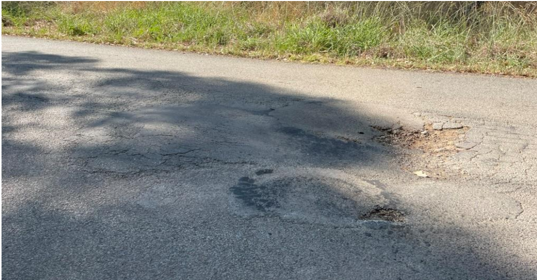
Figure F – Two pavement failures with 'heaves' to their left (Tames Road)
