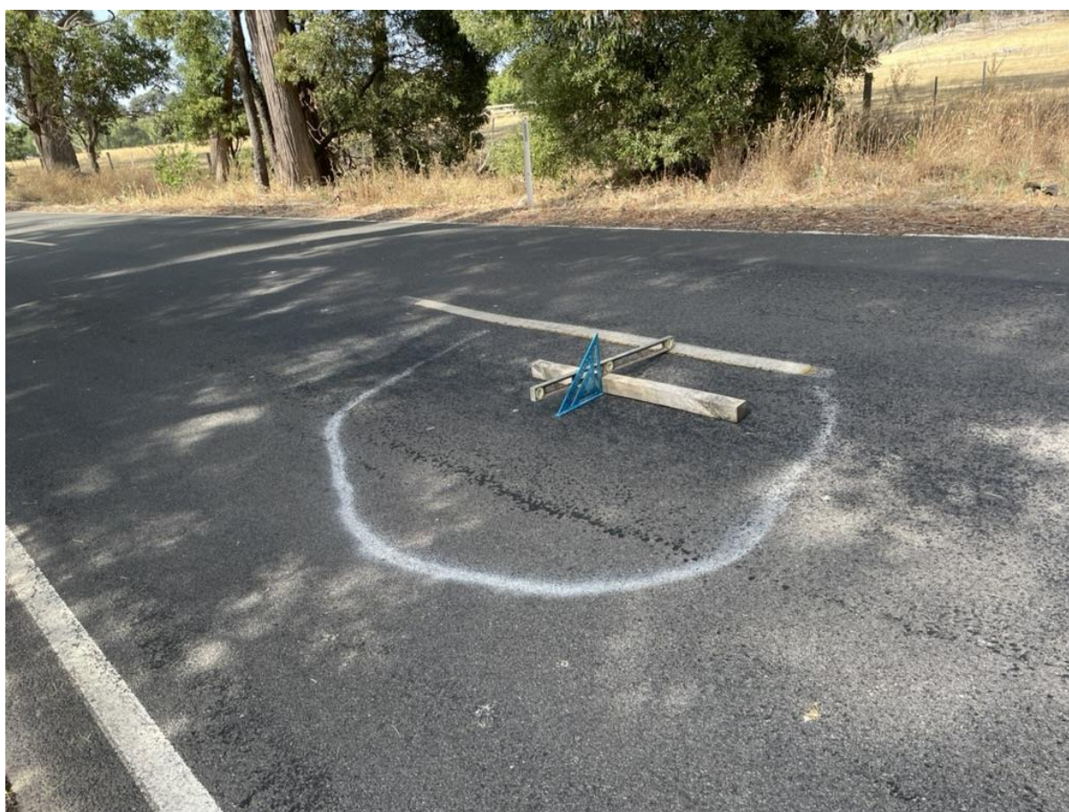
Figure H – Sinkhole along Euroa-Strathbogie Road.
