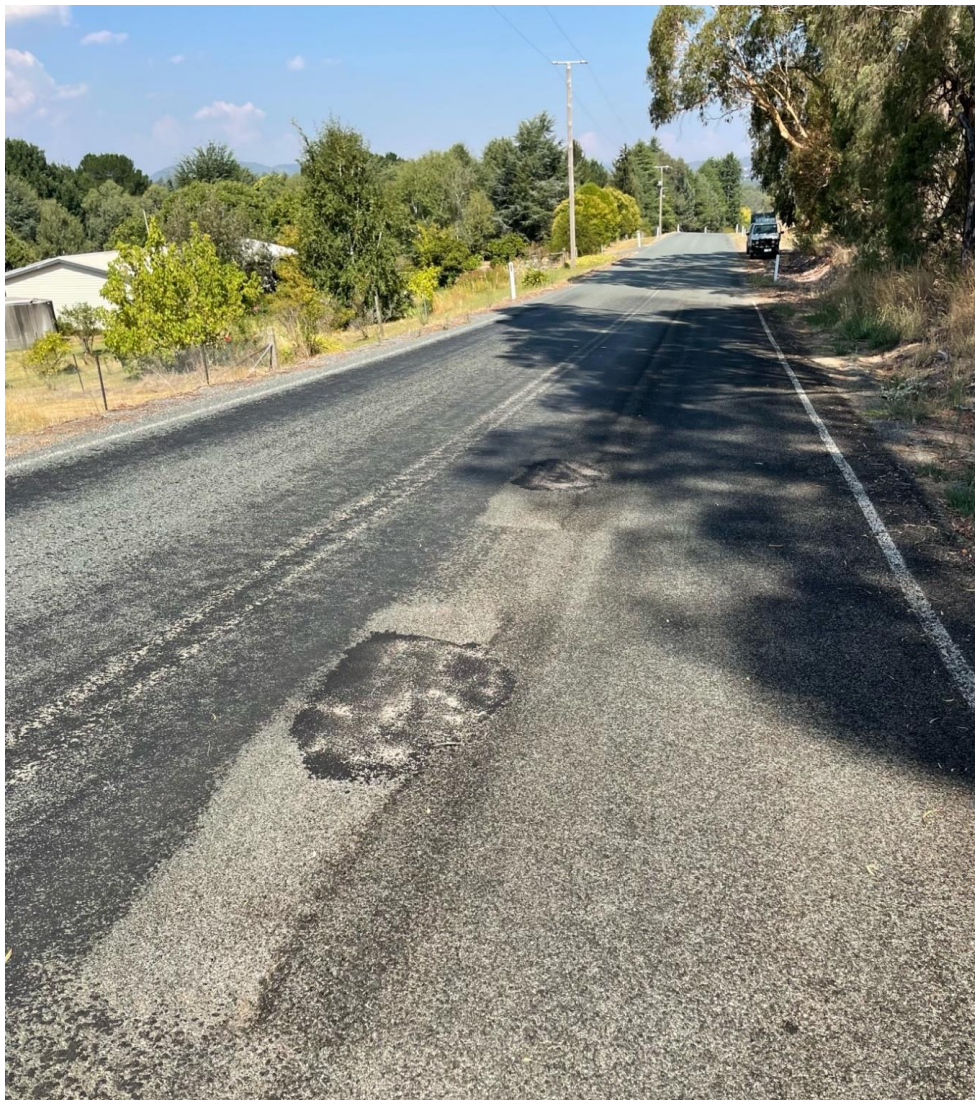
Figure J – Repeated patching requirements on brand new road (Euroa-Strathbogie Road, Strathbogie)
