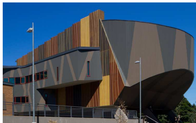
Figure 1: Burrinja Cultural Centre – External view
