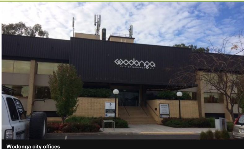
Wodonga city offices
