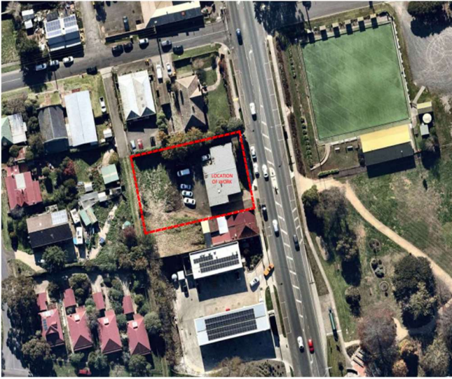
Figure 1 – Aerial shot of project site
