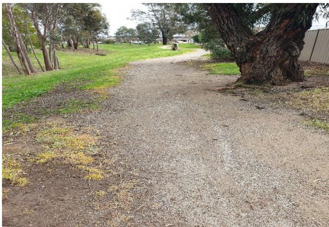
Figure 1 – Taylor's Creek Shared Path – Current conditions (Mitchell Shire Council)
